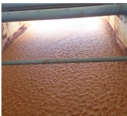
DAF retrofitted with MicroGas™
